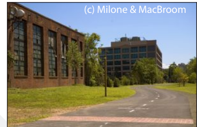
(c) Milone & MacBroom Farmington Canal Greenway
