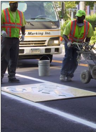
Bike lane installation, New Haven
