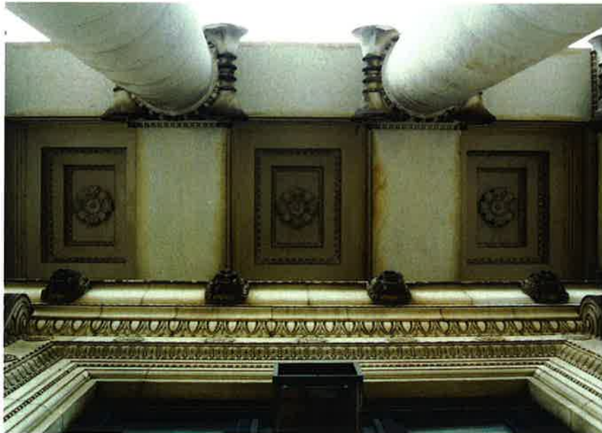
Photograph 21: Ornamented coffered plaster soffit of the portico, south elevation, 2002.
