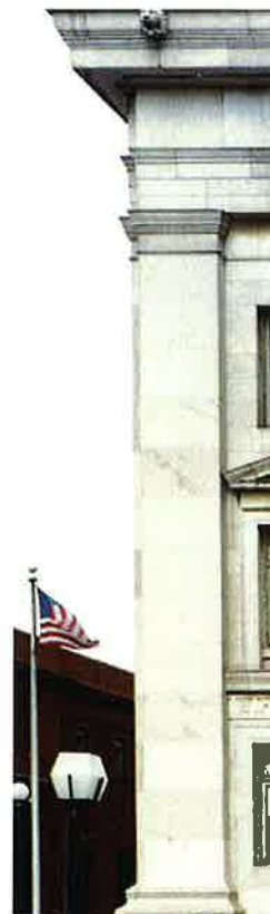
Photograph 11: Pilaster, south elevation, 2002.
