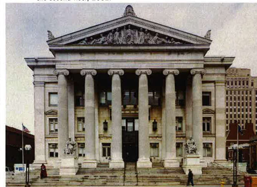
Photograph 17: South elevation, 2002. Photograph by Whitney Cox.
