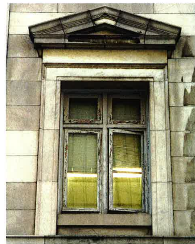
Photograph 16: Paired vertical pivot sash topped by paired awning transom sash framed by an architrave supporting a frieze and cornice surmounted by a pediment, typical for the second floor, 2002.
