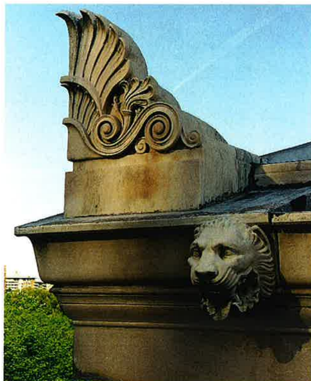
Photograph 13: Cornice from the east elevation ornamented with a lion mask and an acroterion, 2002.
