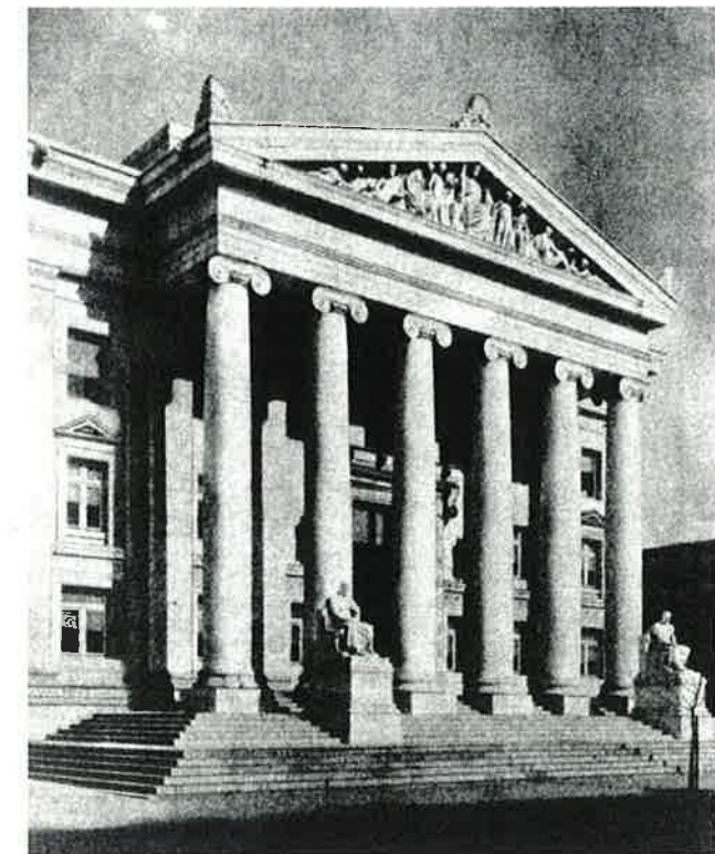
Photograph 10: South elevation showing portico, published in Architectural Record , April 1916.
