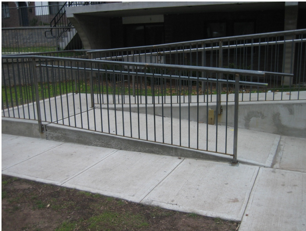
A new handicap ramp was constructed to provide an accessible route to the apartments designated for those with physical disabilities.
