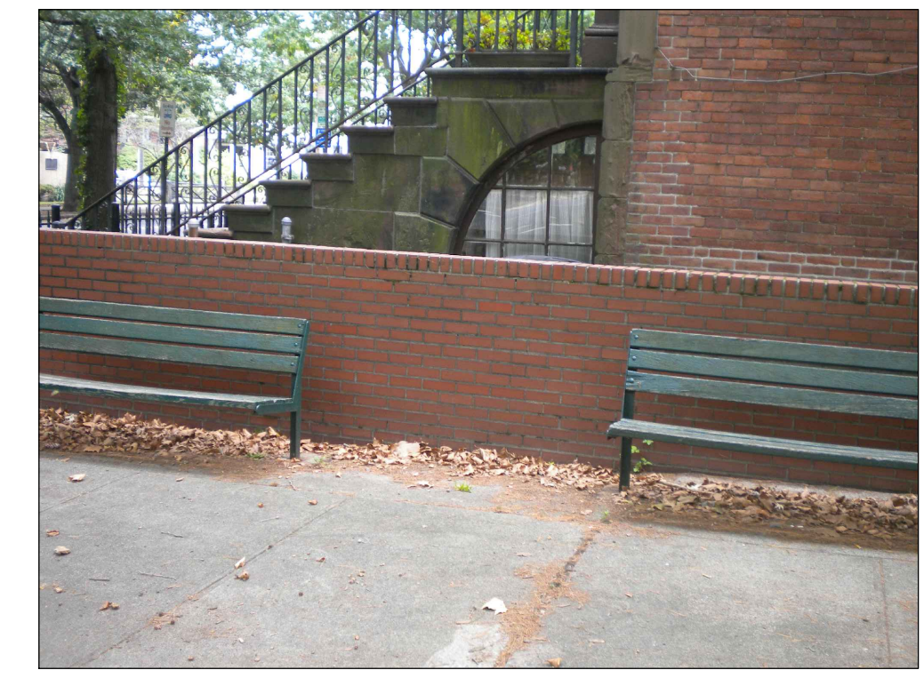
Brick Wall (Existing wall at Russo Park)
