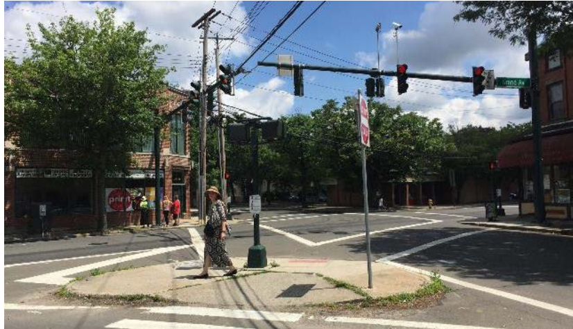
Grand Ave and Olive St intersection could be realigned to minimize pedestrian crossing lengths
