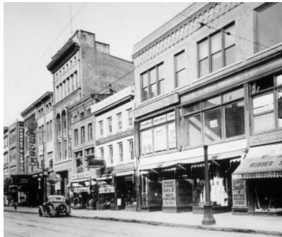
Chapel between Orange and Church, 1933
