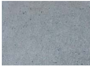
Figure 23 Public Space Paving - Scored Concrete
