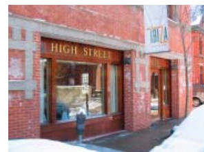
Figure 53 Building sign coordinated with architecture
