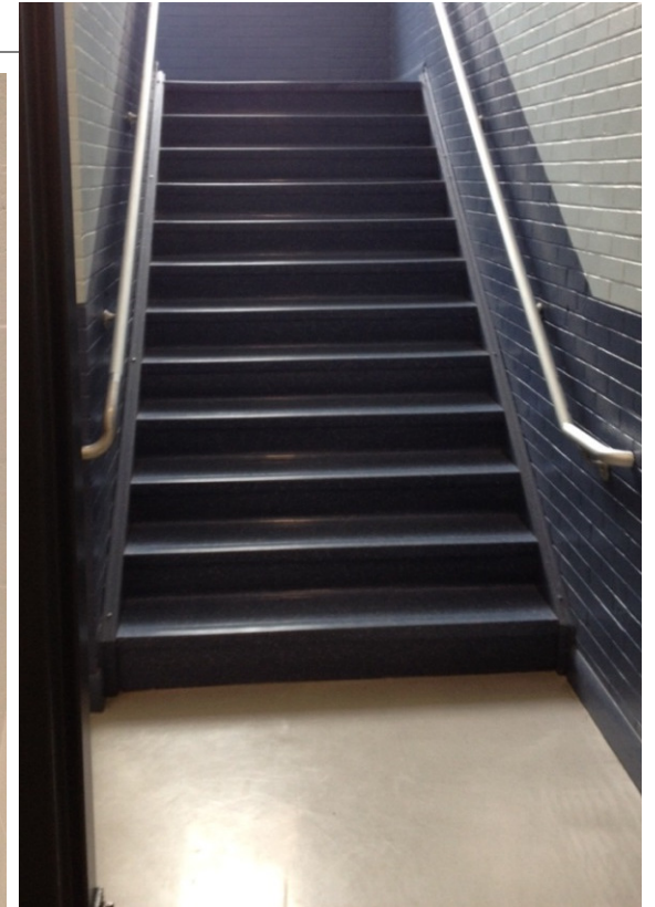
New Stair Treads
