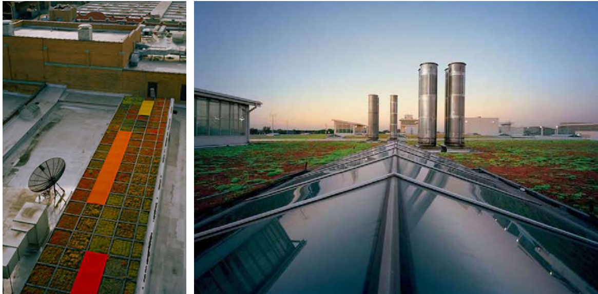
Figure 2. Green roofs over industrial buildings
