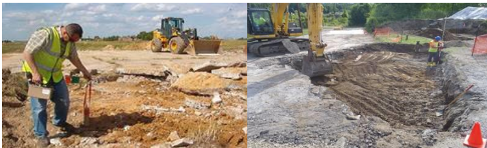
For this project, soils beneath the footprint of the building will be excavated (similar to photos above) and transported off site.
