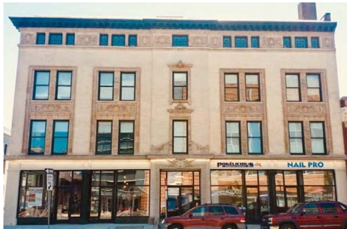
35-39 Church Street | Received a Façade Improvement Grant to restore a historic façade, create two ground-floor retail spaces, and convert the upper floors into apartments.
