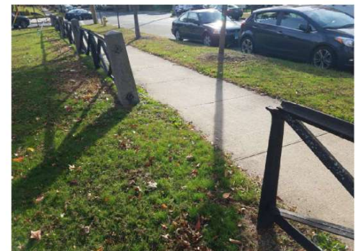
Removed sections of park fencing.
