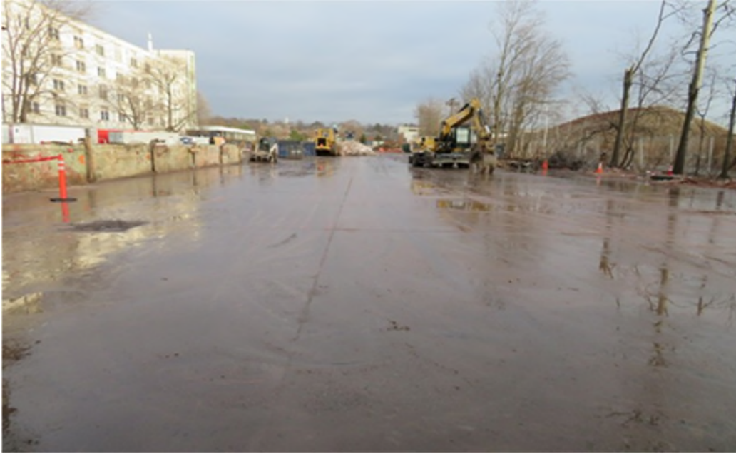
View of concrete slab at column 1 looking east.
