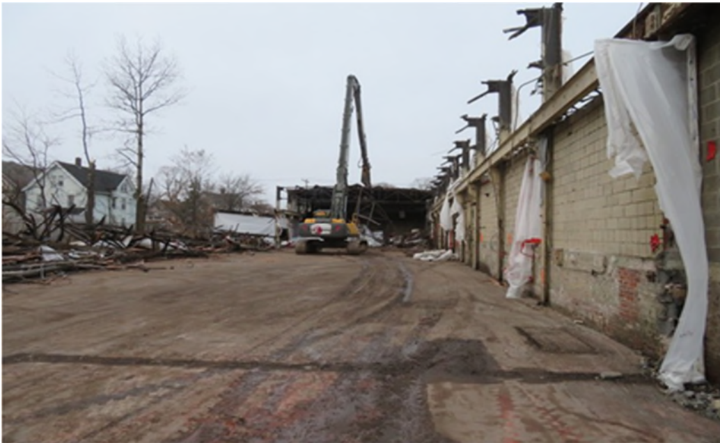
SWC removing steel rafters from columns 14-5.
