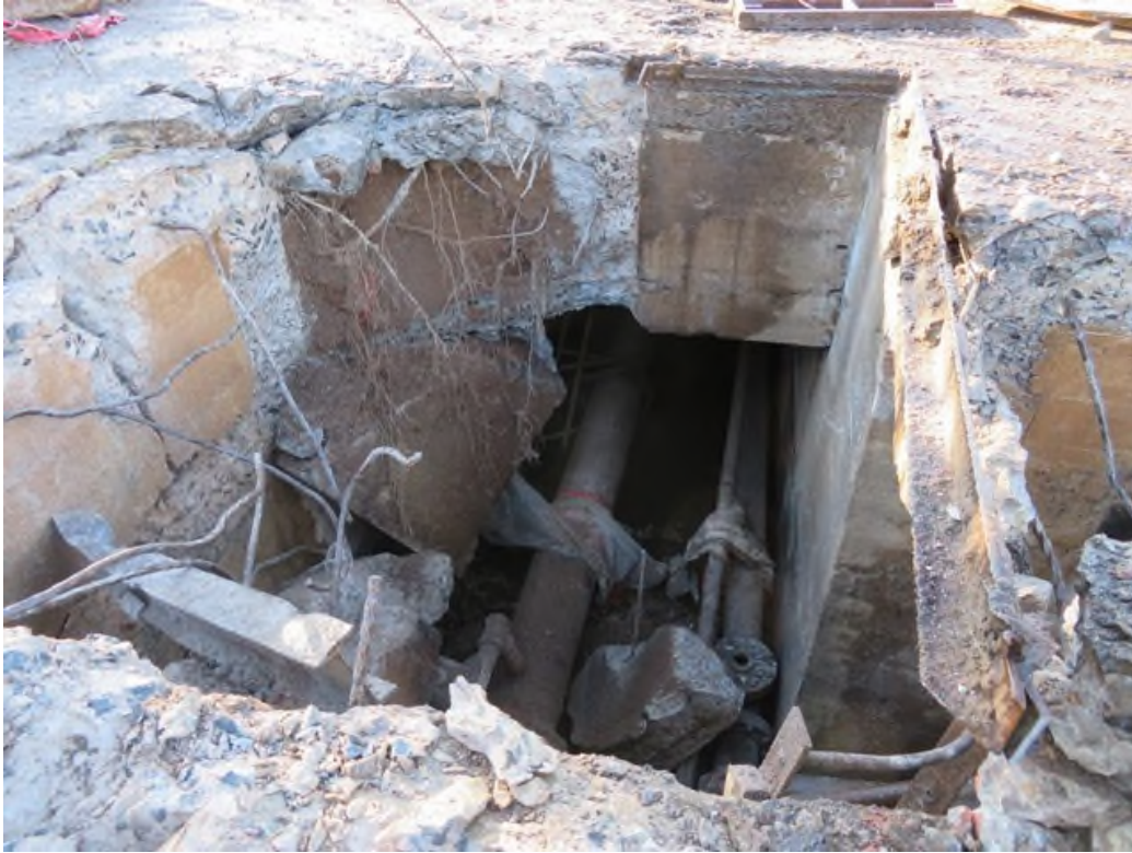
View of deep tunnel looking south towards Argyle St.
