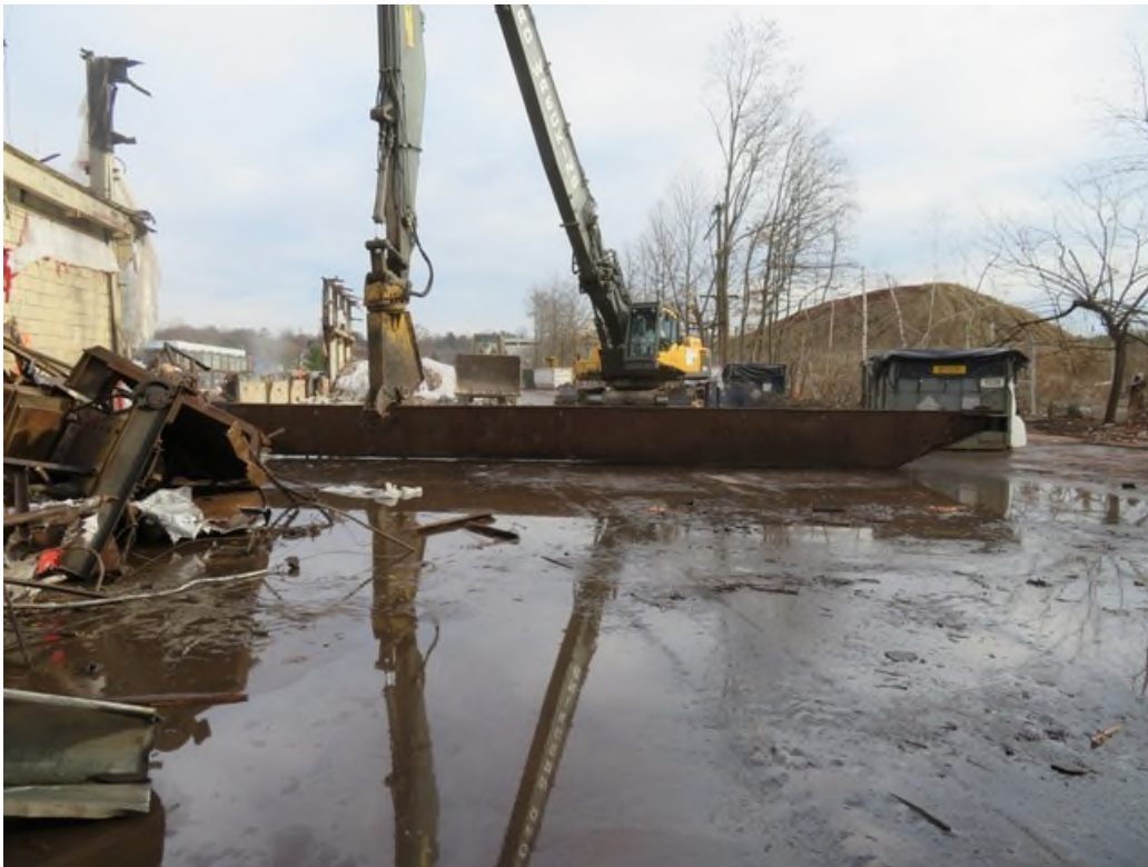
SWC cutting large crane for loadout.
