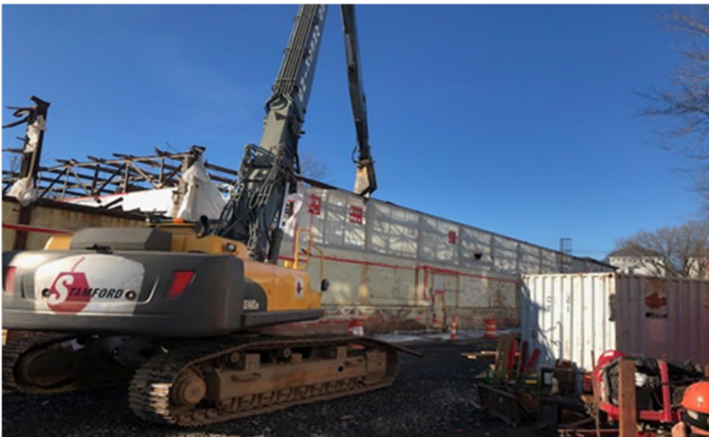
View of window removal.
