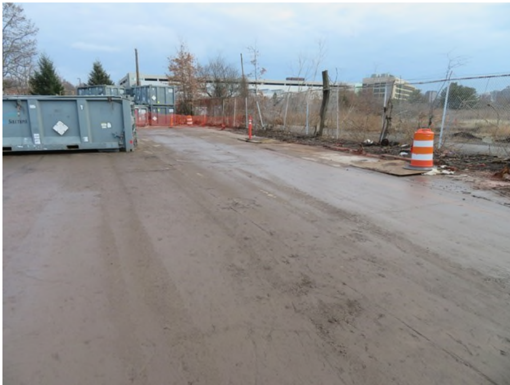
View of slab cleaning.
