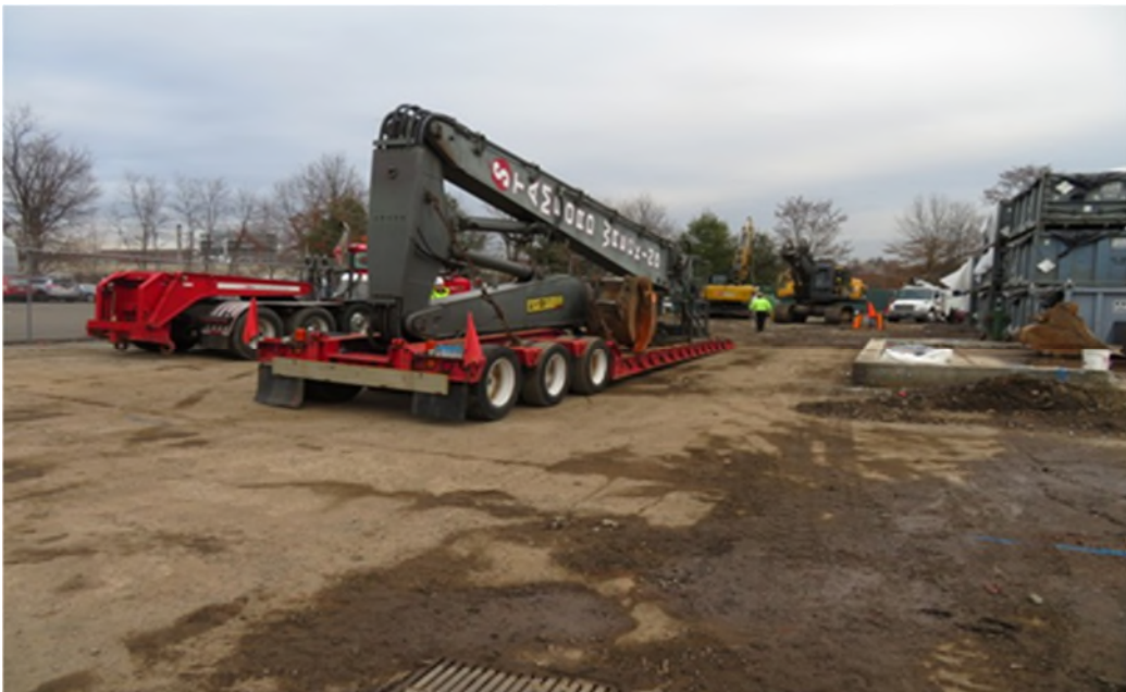
View of high reach excavator being disassembled.
