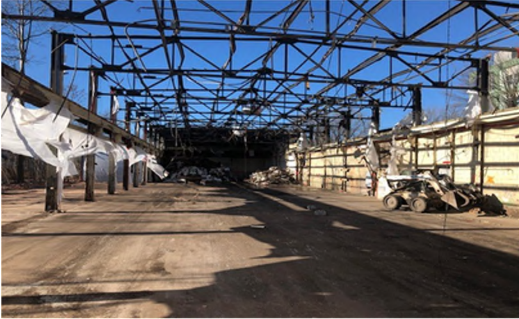
View following window removal.
