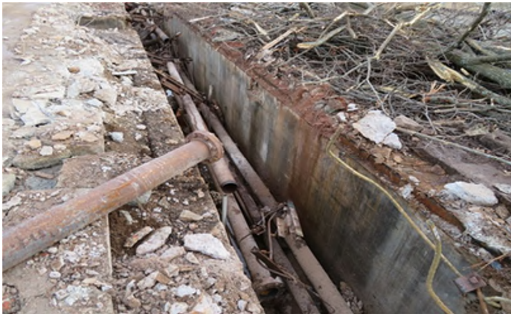
View of pipes inside southern trench.
