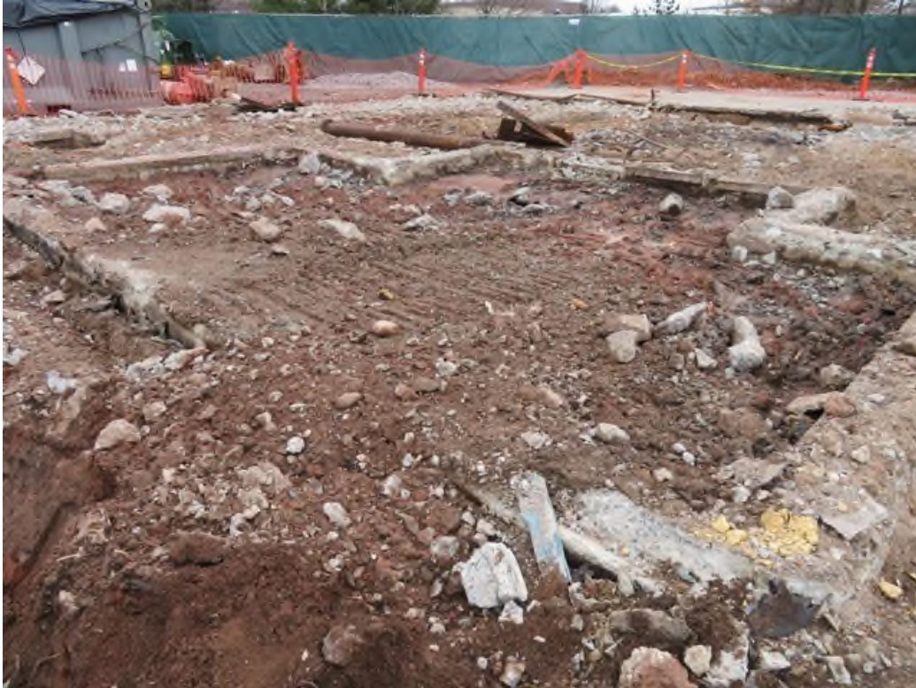
View of interior foundation walls below the slab in Building 3H.
