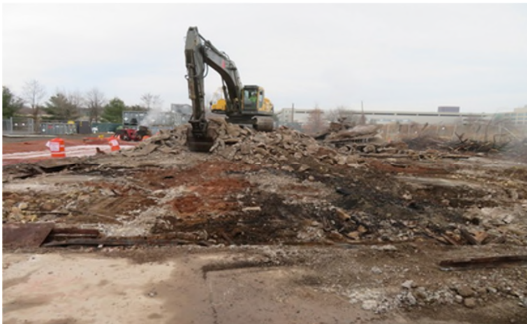
View of concrete slab removal at column 33 looking east.
