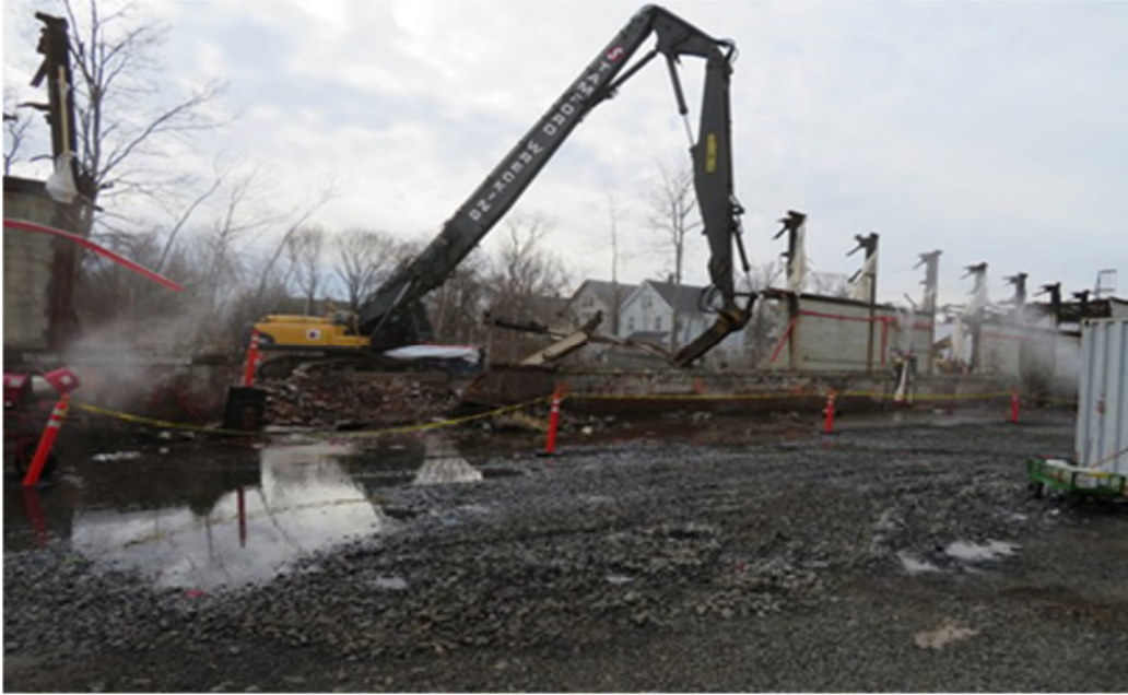
SWC removing northern wall.
