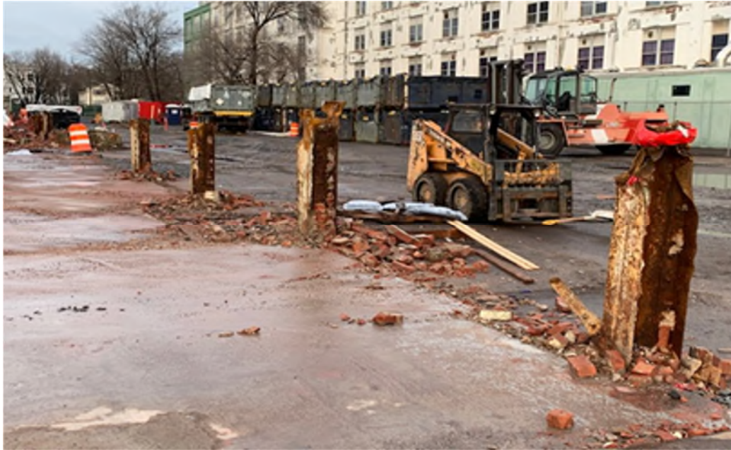
View of SWC removing remaining knee-wall at column 33.
